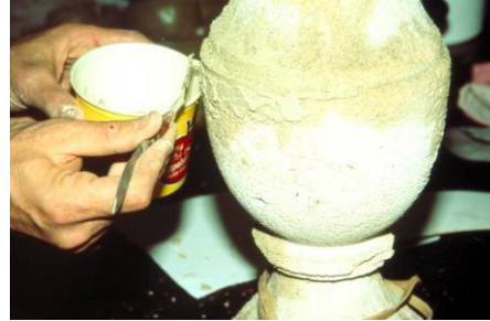
Re-shaping with usual stone-cutter's tools
