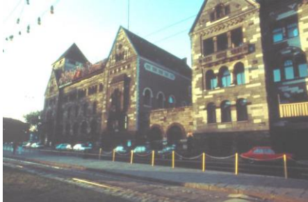
Facade repair by stone replacement
